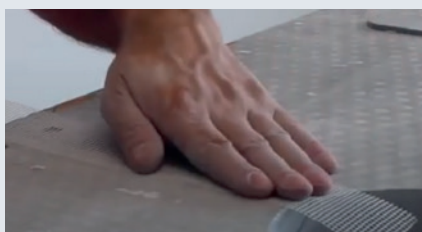
1 Placer Skamol Joint Tape.
